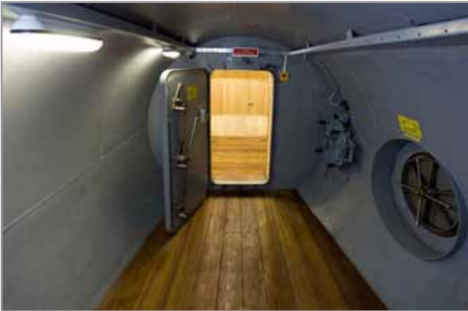
Transfer between the habitable and storage modules. On the right there are lock chambers.
